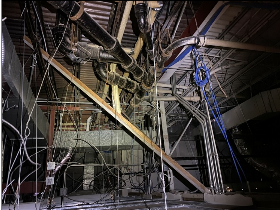
5 - View above the second floor drop ceiling.
