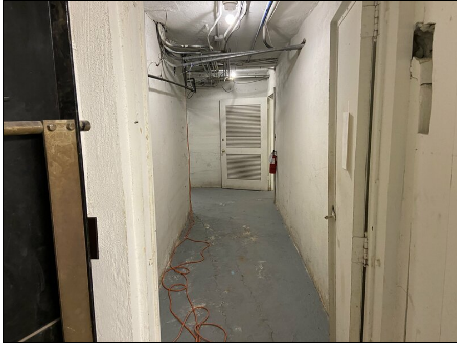
3 - View of basement
