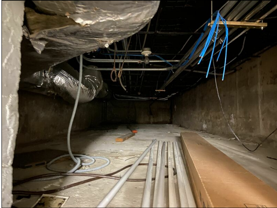
5 - View of crawlspace
