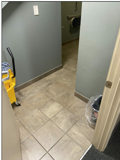
6 - View of first floor bathroom
